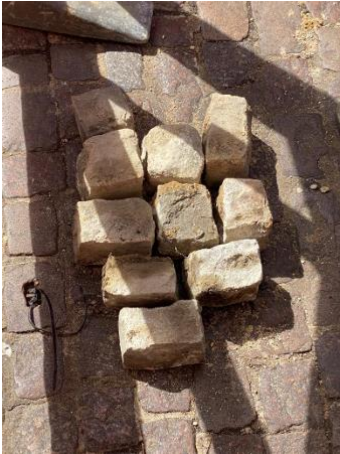
Figure 5: Photo of setts during previous trial pit works
